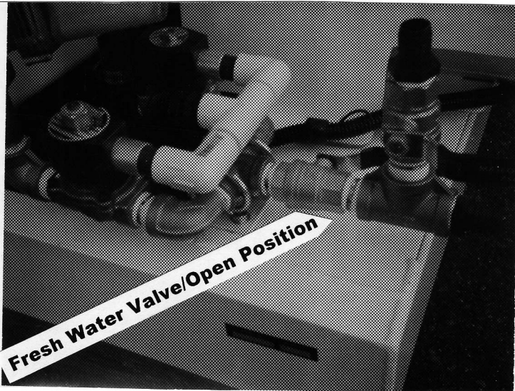
Fresh Water Valve in Open Position:
